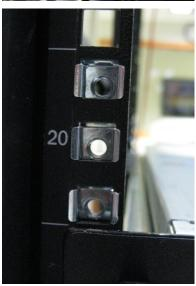
• Attach the rear ear to the cage nuts using the long screws. Please note the orientation of the ear in the photo. The protruding mounting hole should be placed toward the top.
